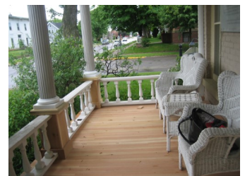
Porch Restoration, Bailey/Lewer House
