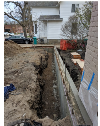
New ramp construction, Bailey/Lewer House
